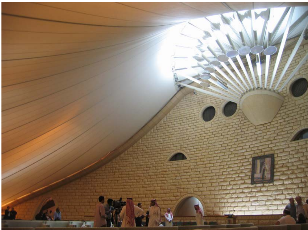
Showing the tent attached to the wall.
