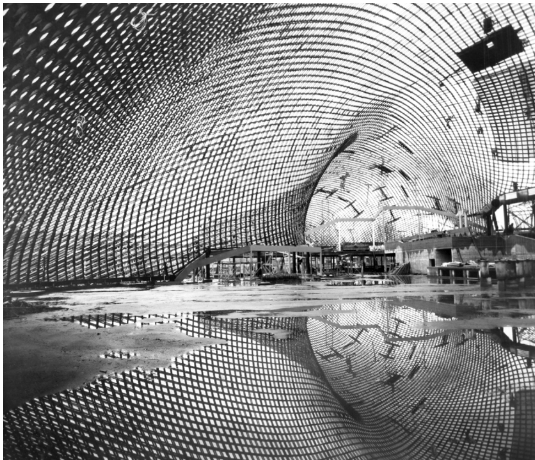
Installing the grid
